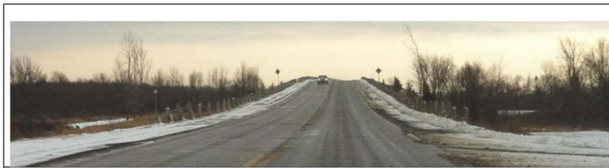
Photo F. Bridge on County Rd 4 crossing the CN Railway.
