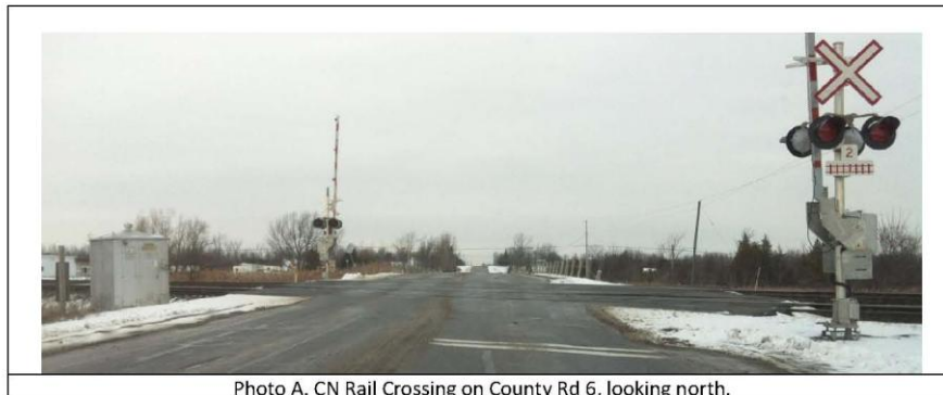
Photo A. CN Rail Crossing on County Rd 6, looking north.
