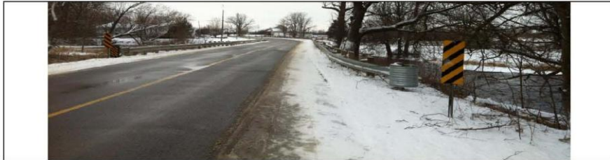
Photo E. Bridge on Millhaven Rd. (looking West)
